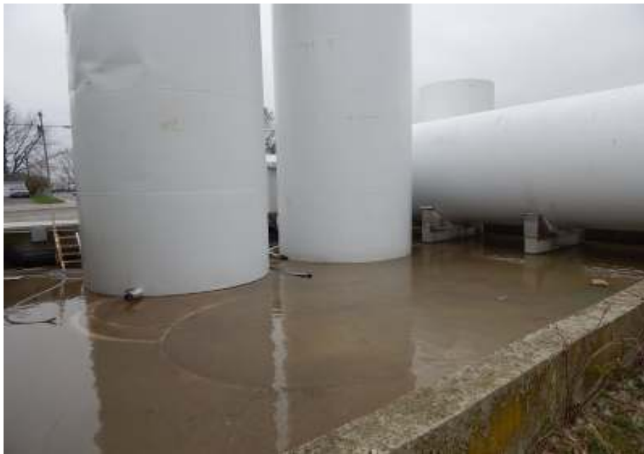
Interior of secondary containment basin. Note rain water accumulated in basin.
